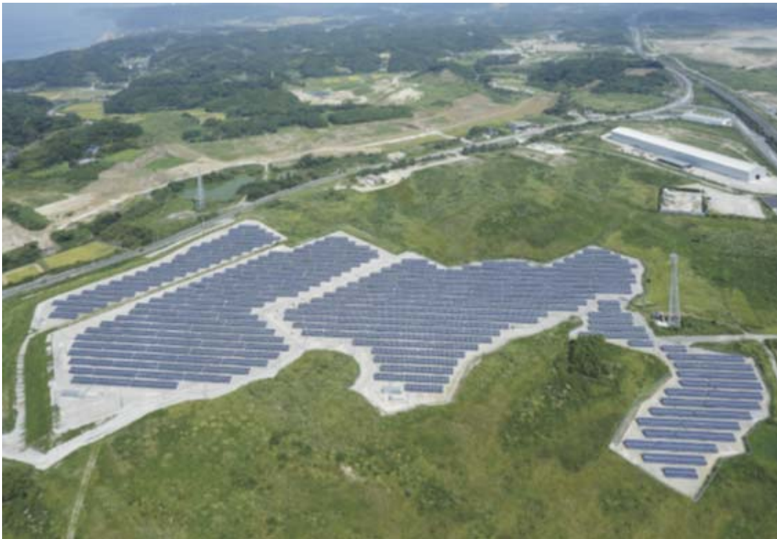
Kasuga Capital Futtsu East Solar Plant • Kasuga Capital Futtsu West Solar Plant
