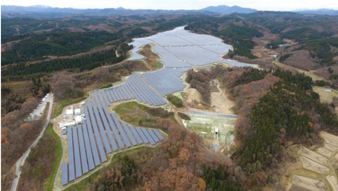
Pacifico Energy Furukawa Mega Solar Plant
