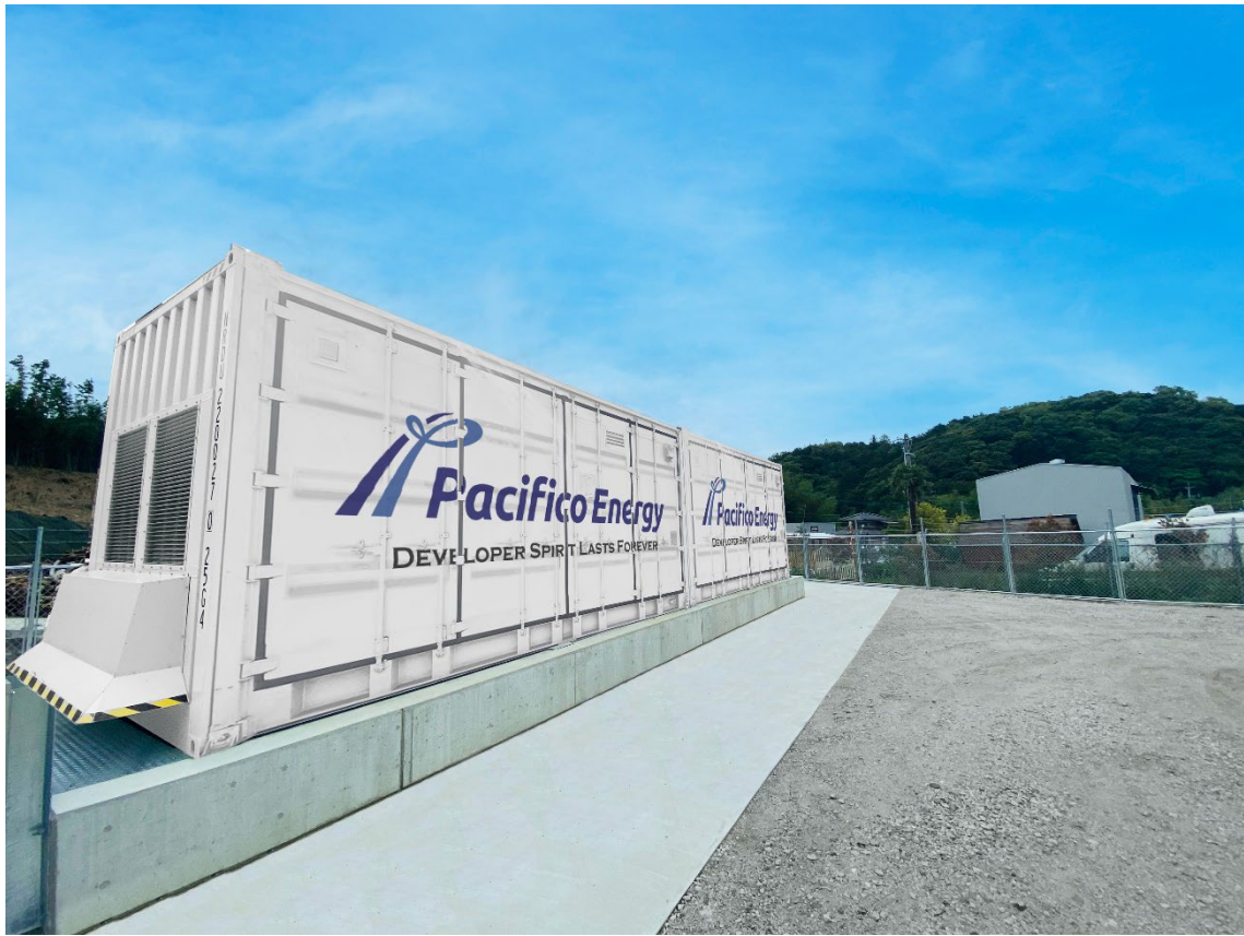
[Installation of Pacific Energy's Shiroishi Energy Storage Plant.]
